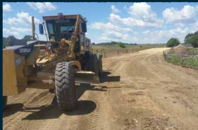
Re-shaping with Grader
