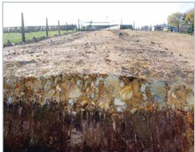
Cross Section of a StockRock™ race.
